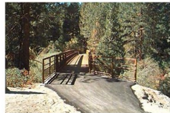
TC5 –Structures frequent or continuous; may include curbs, handrails, trailside amenities, and boardwalks.
